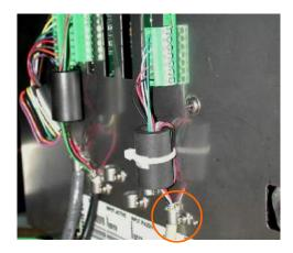
Figure A-22: Shield Wire Termination, Panel Enclosure
